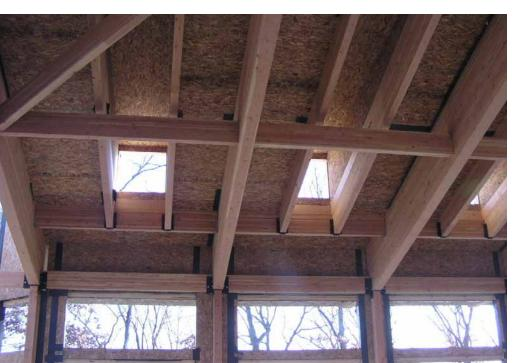
What made SIPs especially attractive to Stromgren for this project was that the SIPs would be fabricated offsite, reducing the framing labor cost. SIP manufacturer Extreme Panel Technologies, based in nearby Cottonwood, Minnesota, used CAD-integrated software and an automated cutting machine to fabricate the panels with exact tolerances. When the panels arrived on the jobsite, the once complicated octagon was reduced to a simple installation.
