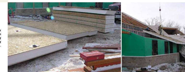
Prefabricated SIPs arrived on the jobsite ready to install, saving time and reducing labor costs. "We were running into problems on the areas with the large windows," said Stromgren. "With conventional framing, the walls would be almost entirely lumber with no insulation. By going with SIPs, we got better wind loading and also increased insulation."
