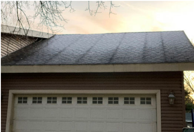
IMAGE 1.3: SIP GARAGE ROOF
