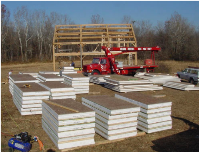
IMAGE 5.6: SIPS STAGED ON JOBSITE
