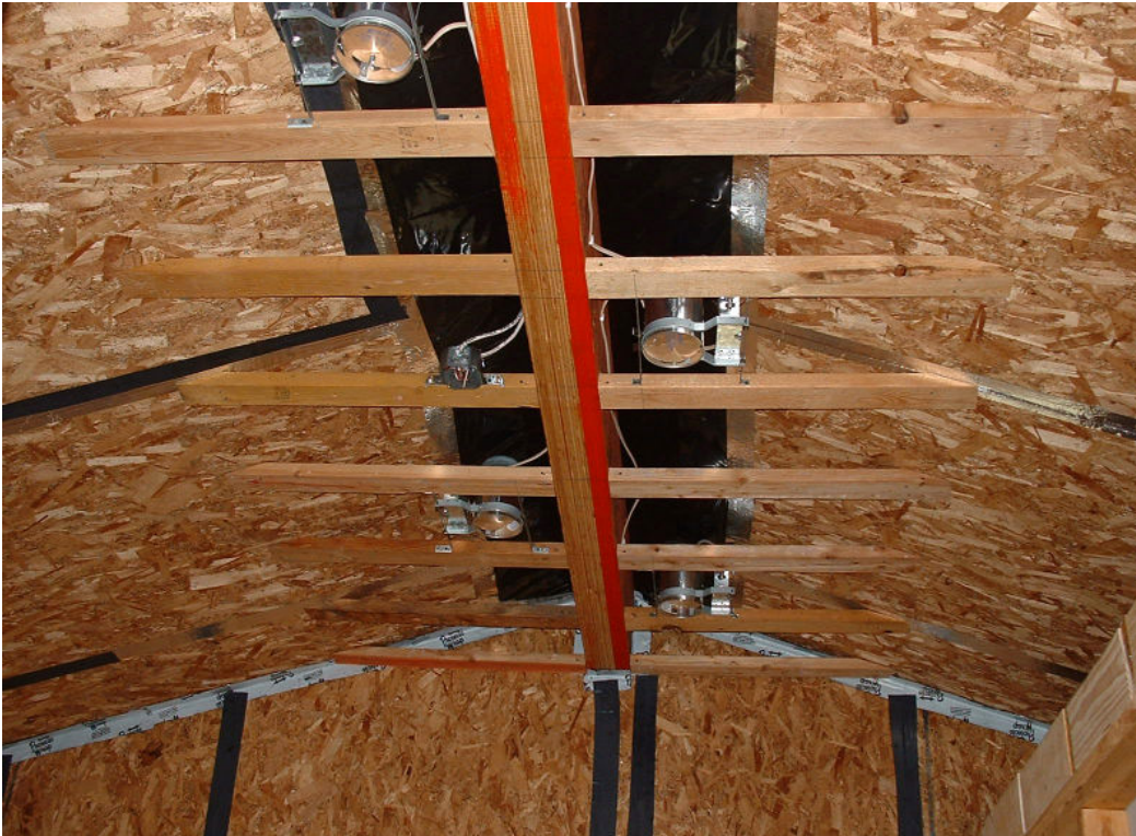
IMAGE 9.8 FURRED-DOWN CEILING FOR CAN LIGHTS
