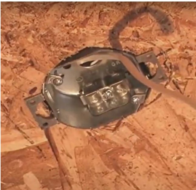
IMAGE 9.5 CEILING BOX INSTALLATION IN SIP ROOF
