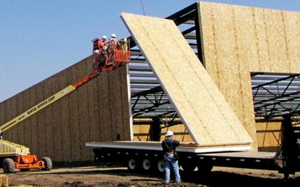
Extreme Panel Technologies has adapted and supercharged the SIPs technology to create both a product and process that yield superior performance.
